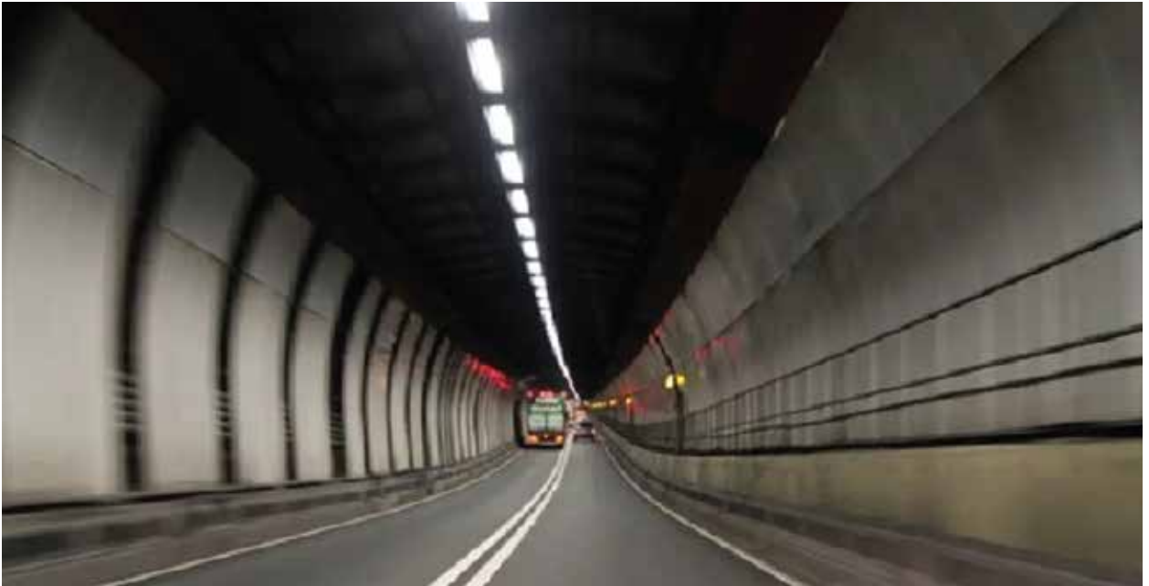
Bangabandhu Tunnel under the Karnaphuli River in Chattogram: One of the 7 Mega Projects that raised questions about their cost effectiveness
